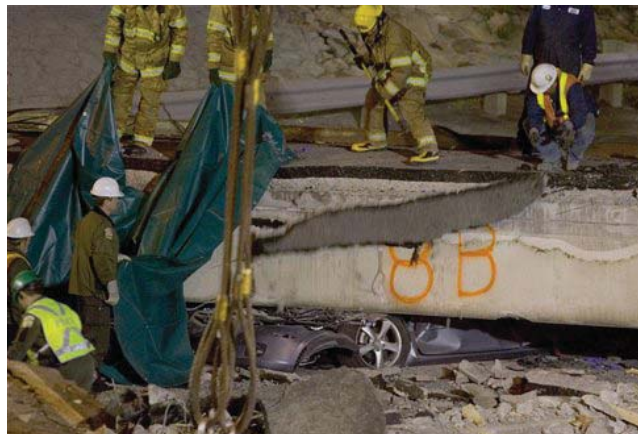
Rescue crews work to remove one of the two flattened cars after an overpass collapsed in the Laval suburb of Montreal, Canada Saturday, Sept. 30, 2006. Quebec provincial police said Sunday that at least five people were crushed to death in their cars after the collapse of an overpass near Montreal. (AP Photo/Montreal le Devoir via CP/Jacques Nadeau)
